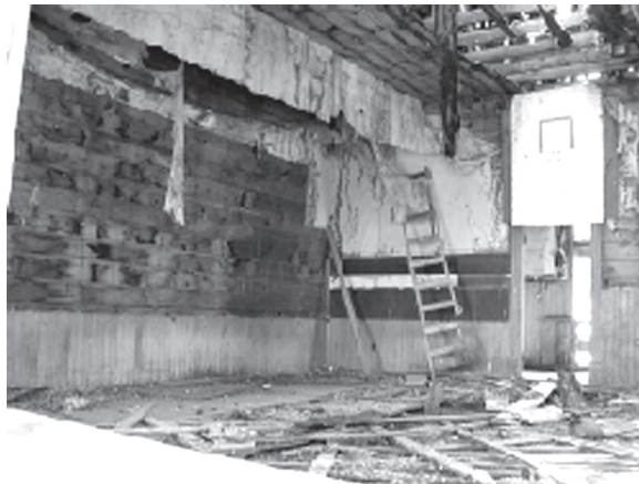
View of Mt. Glen School classroom in 2002, as seen through rear window frame (no glass in windows; roof in disrepair; floors in poor condition.) Photo by Eugene Smith
